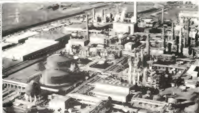
The Great Plains Coal Gasification Project near Bismarck, N. Dak., is slated to receive federal funds
